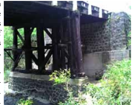
Nīnole Bridge, near Punalu'u, will be replaced. Photo from DOT
