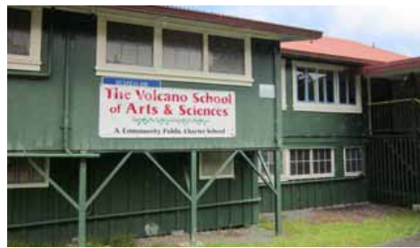
Gov. Abercrombie has released funds for new buildings at VSAS' Keakealani Outdoor Education Center campus.
