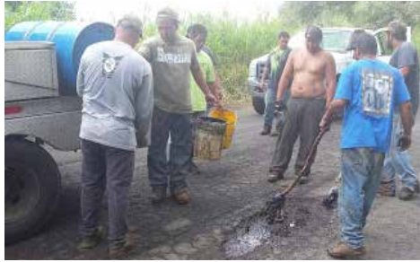
Crewmembers fill potholes on Ka'alaiki Road. Photo by Davelyn Barido
