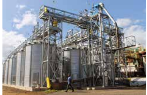
New drying towers for Royal Hawaiian Orchards macadamia in Pāhala.
